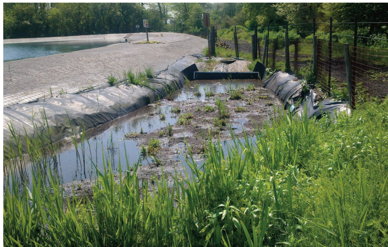
Bordon Hill continues to expand their reed beds, which filter runoff water from the facility and prevent nutrients from leaching into the ground and surface water.
